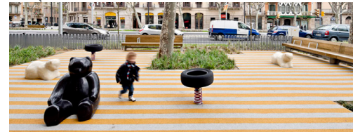
The playground will be with prefabricated pavement with draining joints which are going to be laid down.
